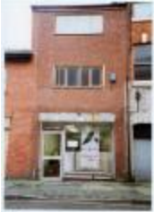
Photograph '1998-1999 Fire - shop unit in construction' (GB3451/OC/5/1/1)
